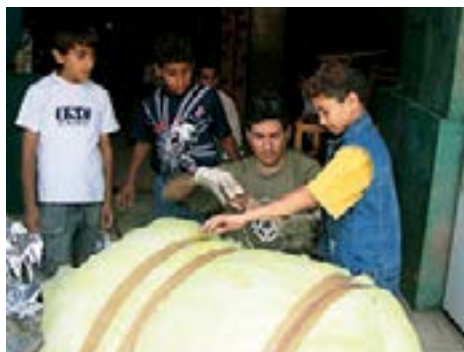
▲ With insulation, the water tank will not lose its heat as fast.
