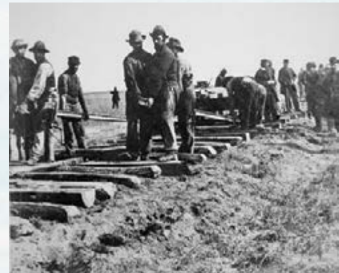
▲ Workers lay new track for the railroad.
